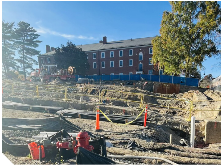
Union TENS installation at Smith College, Massachusetts
